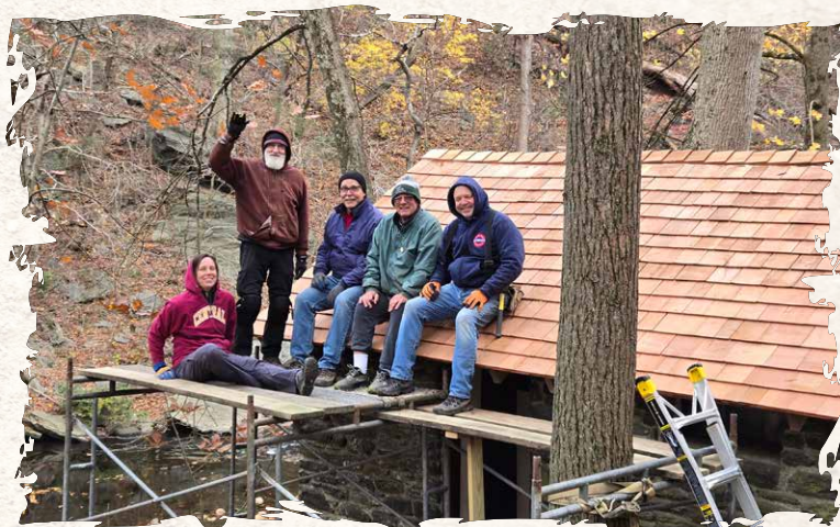
FOW's longest-running trained volunteer group, the Structures Crew, repaired the Kitchen's Lane structure this year to its original glory. Photo by FOW staff
